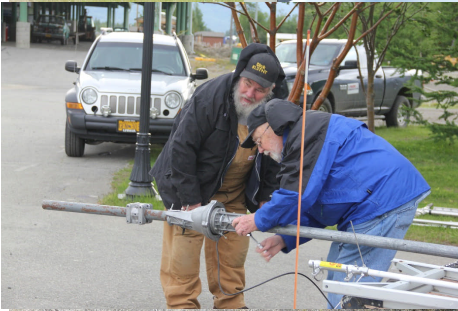
EXTEND MAST AND SECURE & INSTALL ROTOR, ORIENT IT NORTH, INSTALL ROPE ON YARD ARM FOR G5RV
